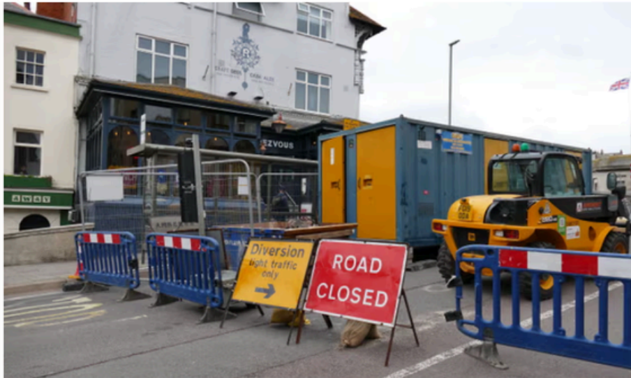
For a long time, construction was overlooked as an air pollution problem by both government and scientists. Photograph: Geoffrey Swaine/Rex/Shutterstock
