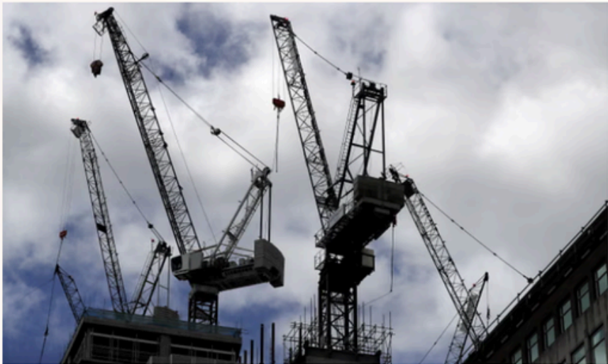
Construction cranes in London. Photograph: Kirsty Wigglesworth/AP
